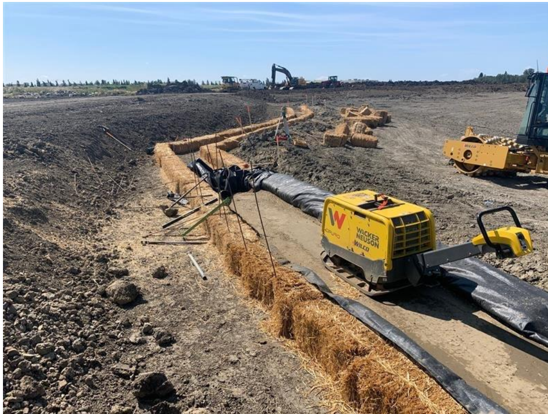
Jensen Lakes Progress Pictures August 14, 2020
