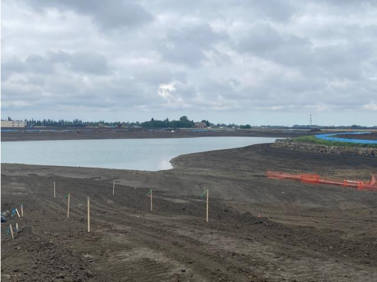
Progress Pictures June 11, 2021
