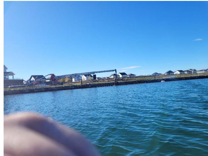
Workers placing gravel along southeast shore.
